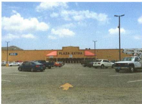
Front exterior of improvements (Photo Taken on June 16, 2015)
